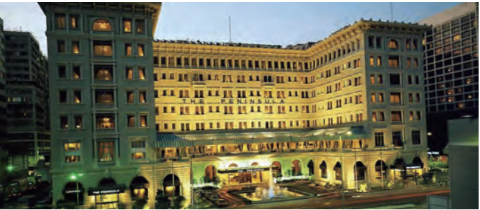
30階建てのタワー建設前 ©The Hong Kong Heritage Project_Creator:The Hongkong and Shanghai Hotels Limited
